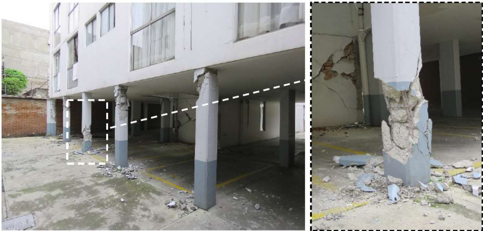
Figure 10. Shear failures in columns in a RC flat slab building with a soft first story at Paz Montes de Oca 93, Col. Gral Anaya (photos by Pablo Heresi).
